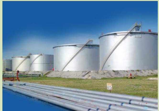
Petrojam Storage Tanks
