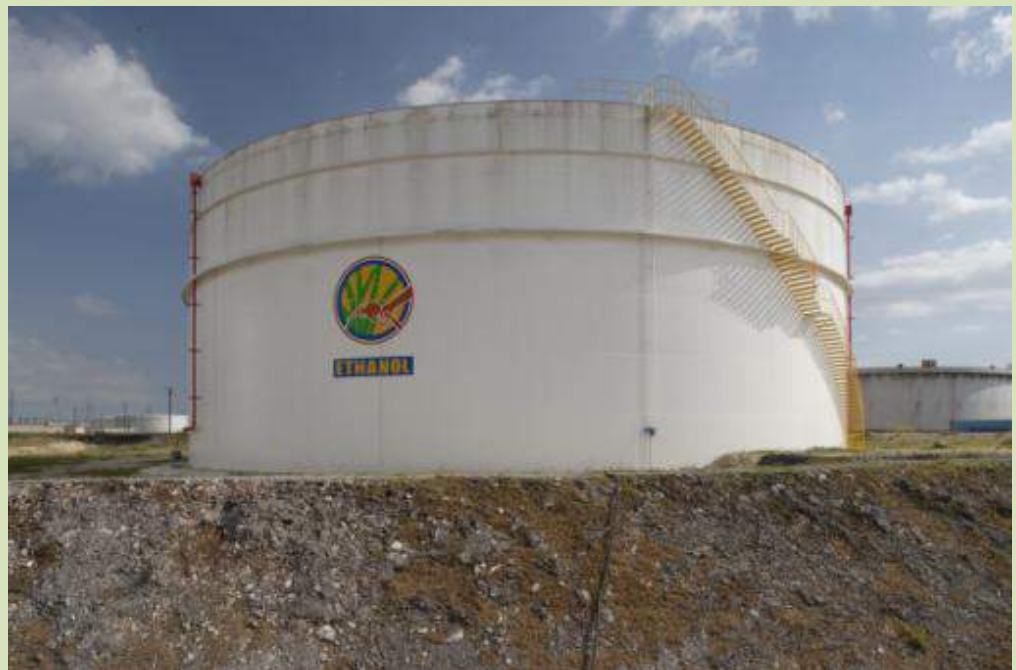
Petrojam Ethanol Storage Tank
