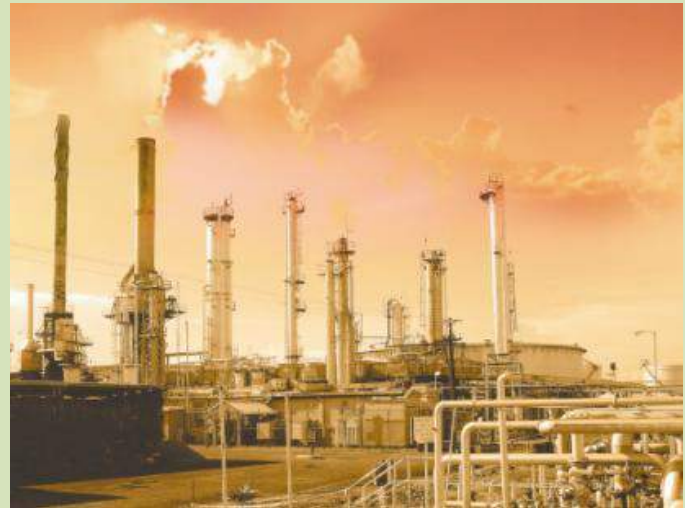
PETROJAM Oil Refinery
